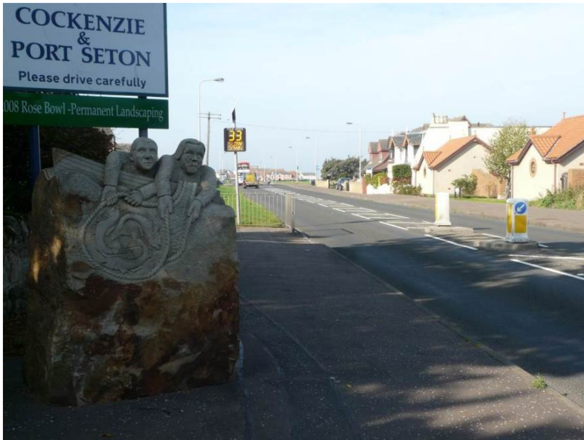
Figure 8.15 Threshold treatment with identity feature, median island, and vehicle activated speed feedback sign - Source: Dr Peter Cairney.
