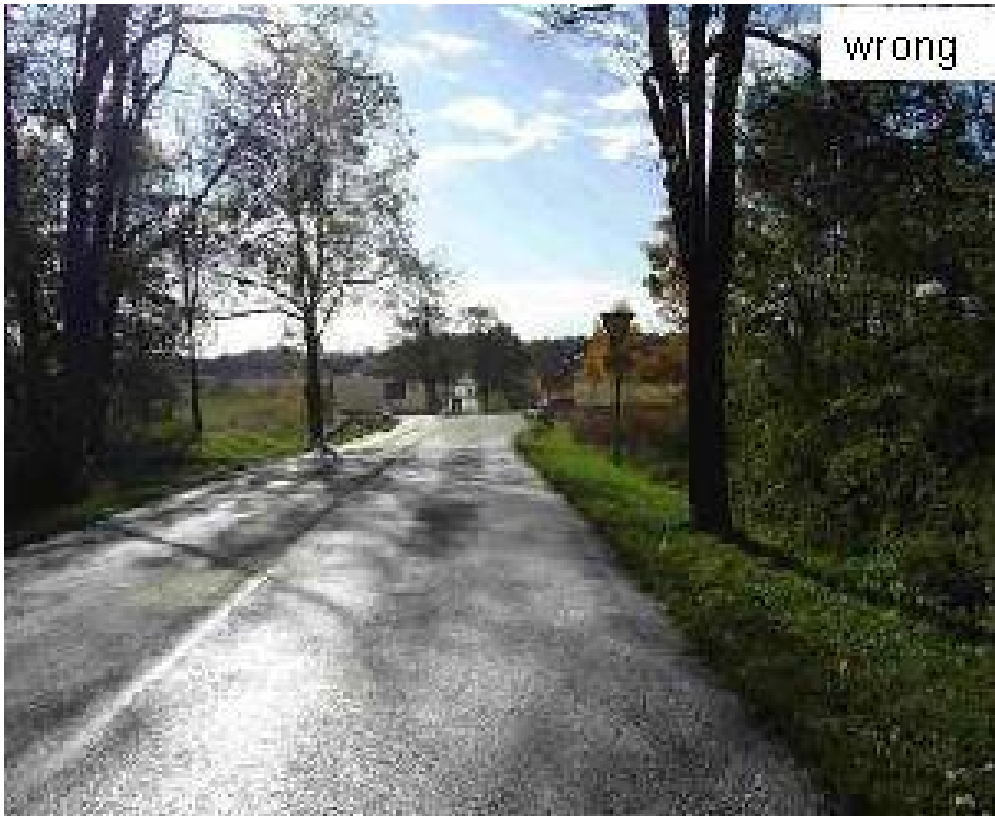
Figure 8.4 Intersection not visible 125 m ahead: unexpected braking and high speed cause of rear-end collisions (Source: Birth, Sieber, and Stadt, 2004)
