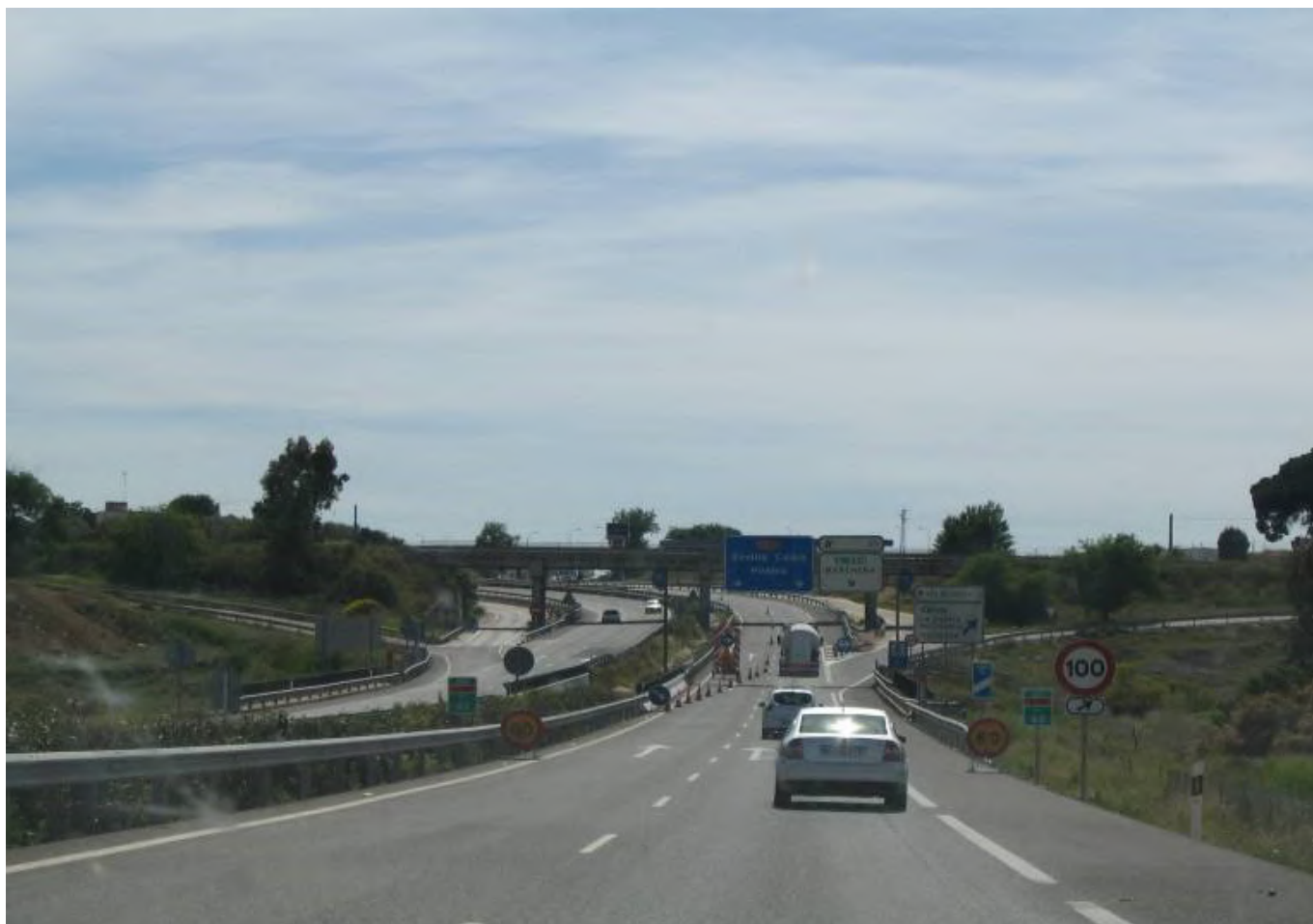
Figure 8.14 Three critical locations: maintenance point, starting a curve and exit road without transition and/or progressive information (150 m ahead) (Birth, et. al, 2006)
