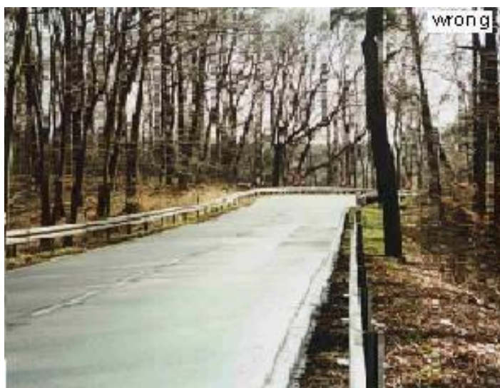
Figure 8.15 Three oversized chevron signs in red and white are not visible against the background in an accident curve (Birth, et. al, 2006)
